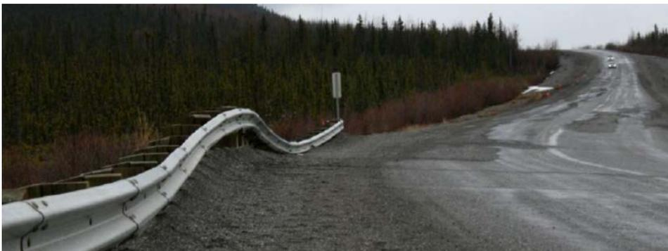
[Differential thaw-settlement of a highway caused by degrading permafrost.](#)
