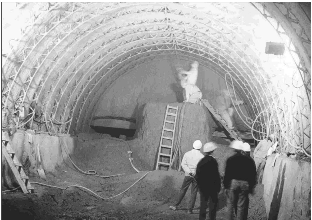
Fig. 2. German Method of tunneling and first use of shotcrete, Line B, 1998.
