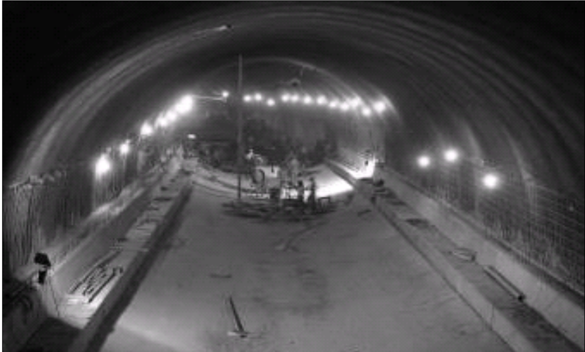
Fig. 7. Tunnel after placement of the invert, Line B.
