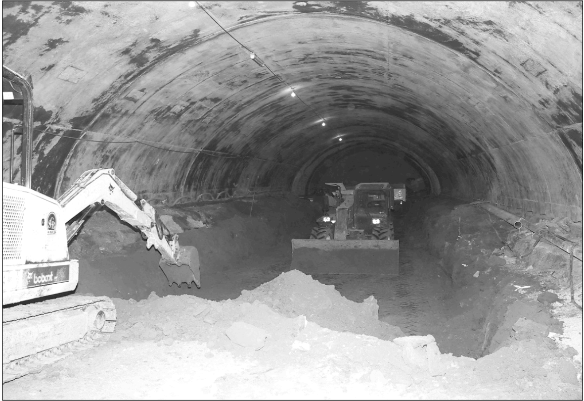
Fig. 3. "Belgian" tunneling method, Line H, 2000.
