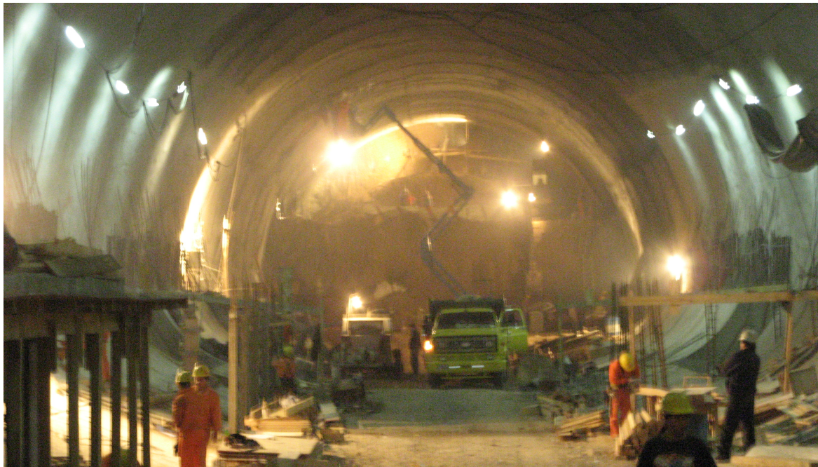
Fig. 9. Corrientes Station, Line H. Full face excavation.
