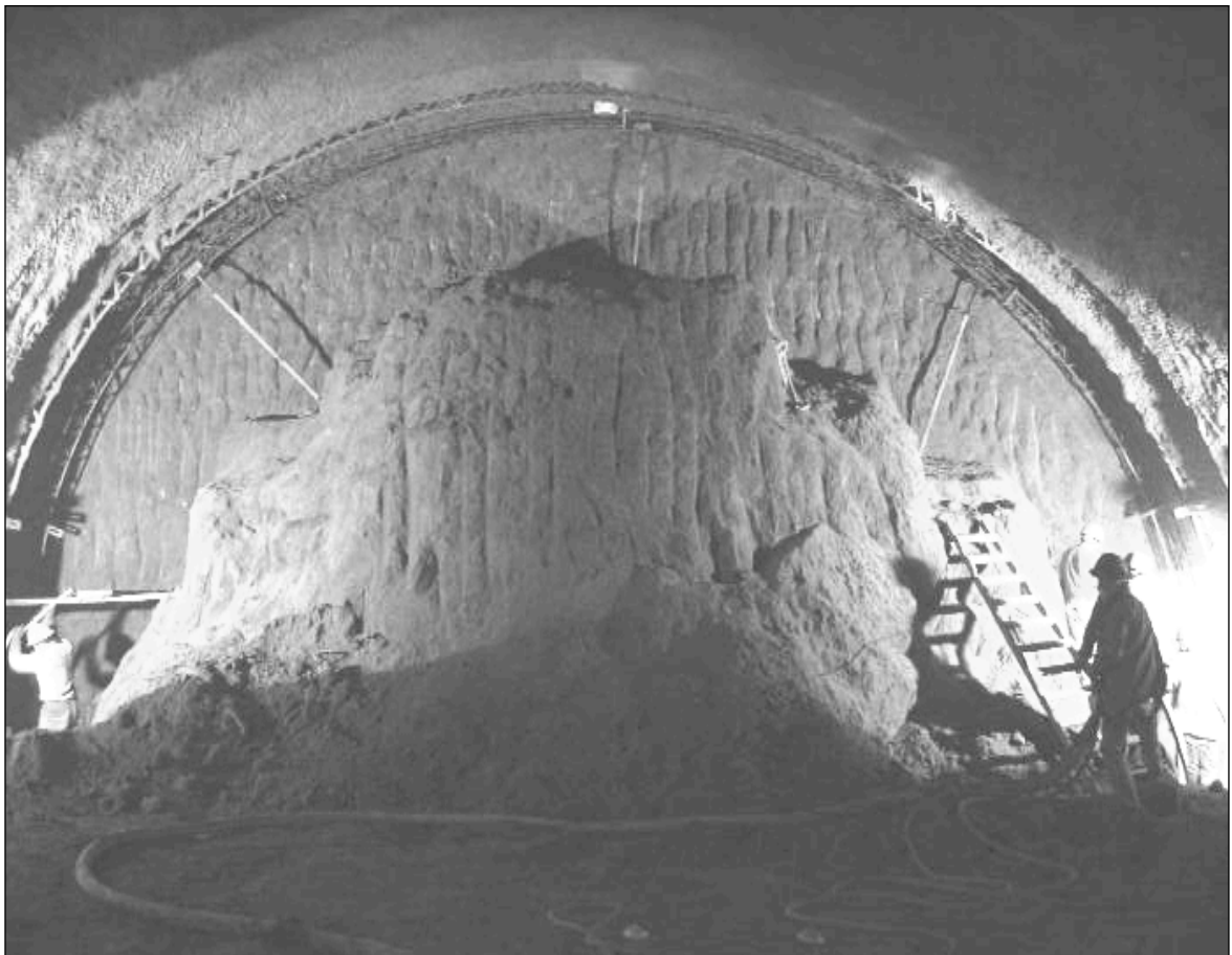
Fig. 4. Full face excavation, Line B, 2004.
