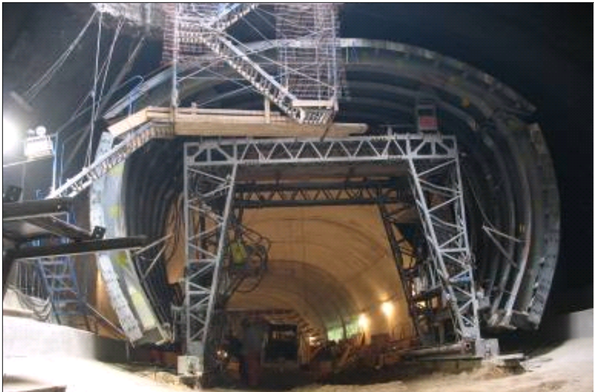
Fig. 8. Formwork used to cast the secondary lining, Line B.
