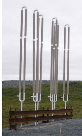
*A thermosyphon-based design was predicted to provide more immediate and dependable ground cooling to stabilize the permafrost and massive ground ice with a more predictable project schedule and acceptable costs.*
