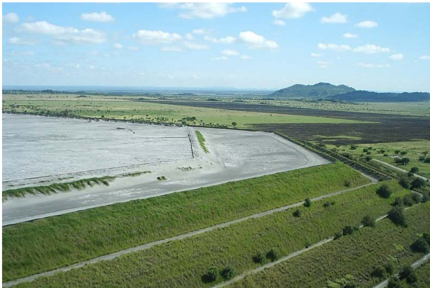
Continuous efforts are taking place to find ways of making tailings storage facilities safer. Image credit: SRK
