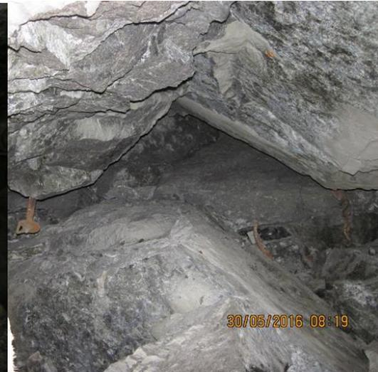
Stress Damage (depth of failure)
